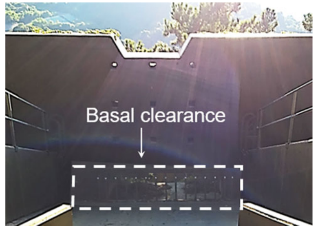
Fig. 2 Basal clearance under a rigid barrier (Tung Chung, Hong Kong)
